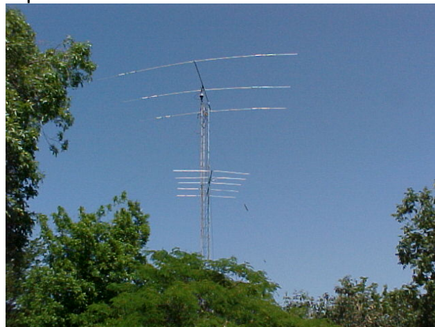
Tower #2, tri-bander and 6 meter beams
