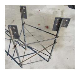
The mounting plates were punched at a steel company and welded to the heavy rebar by a certified welder (not me). After attaching the plate assemblies to the tower, Pieces of rebar were welded to keep the shape during the cement pour.
