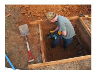
The hole required a 20-pound jack hammer and a son who works for food. Wilton soil is only slightly less hard than the cement. The 2X4 frame in this shape allows it to he secured with construction stakes without making the sides crumble into the hole.
