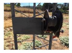
After cranking down the tower, removing the cable from the winch and removing the winch from the tower plate I could install the shelf to determine where I needed to drill two holes on the left of the tower plate. There are a total of five bolts holding the shelf to the tower plate.
