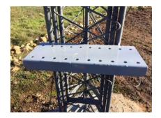
After getting the shelf level and installed it was a simple matter to install the winch on the shelf. Before bolting it down to the shelf though I had to take the hoist motor/reel off its frame to install the tower cable.
