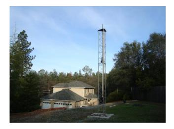
Earlier this week, Fred, K6IJ and I installed the Rohn 45 top section, thrust bearing and T2X AZ rotor for the 6M EME array. I will be checking out the M2 MT-3000A elevation system next week, and hope to get it installed on top the tower before the end of the month.
